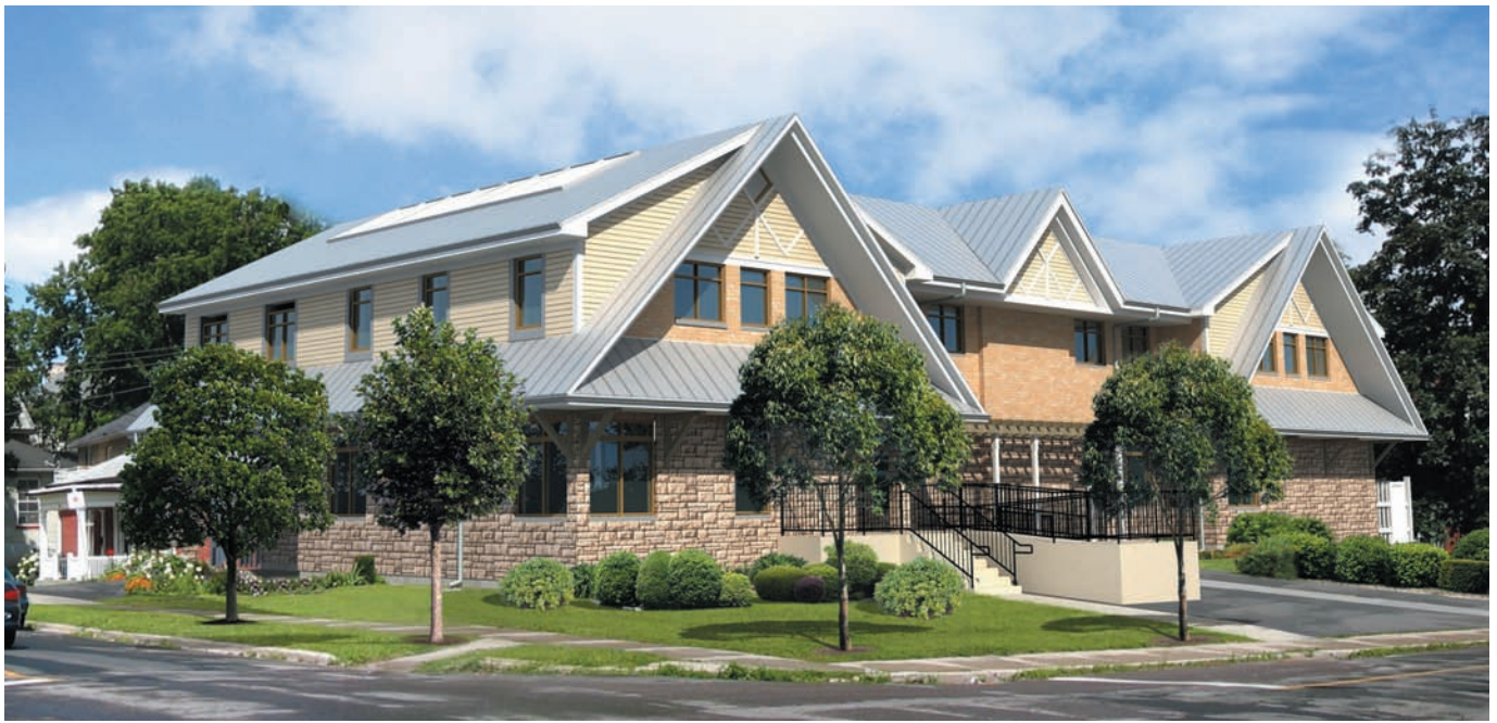
New YWCA Crossroads Safe Haven Shelter. Image created by Trevelyan Architect Inc.
